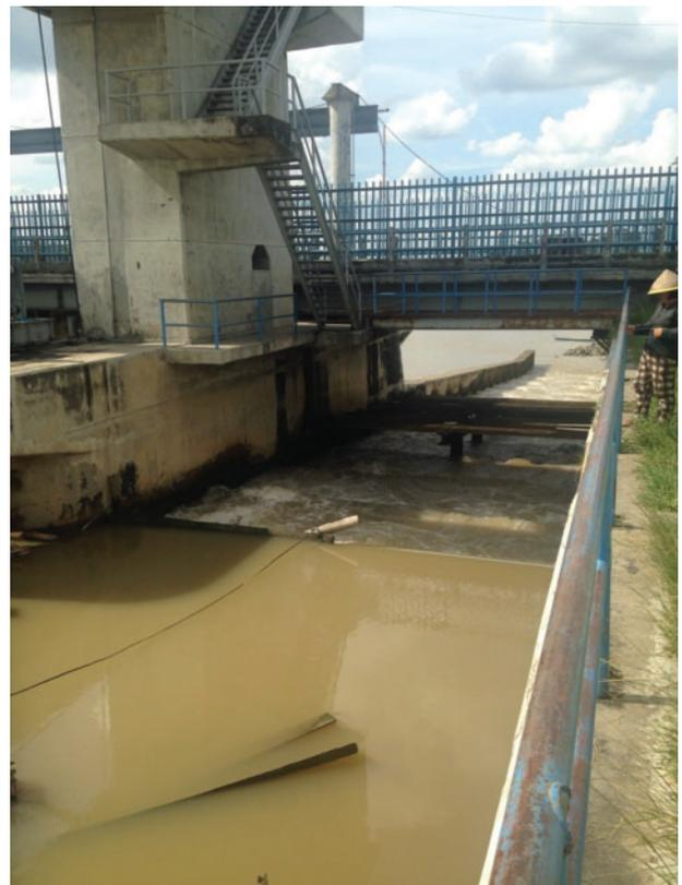
**Fig. 3.** Close up view of Perjaya fishway, demonstrating that both fishing nets located downstream of the fishway exit and the location of the entrance significantly downstream of the regulator gates.
