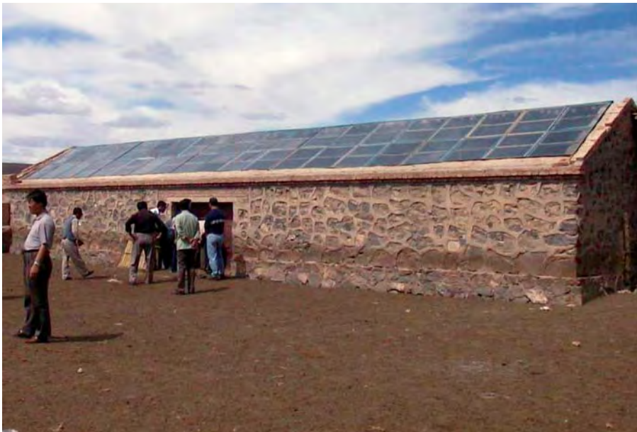
An example of a new warm shed (note the clear plastic roof) in the Inner Mongolia Autonomous Region. Holding animals at higher temperatures during winter reduces their weight loss. [Photo: D.R. Kemp]
