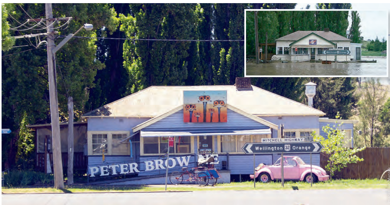
Flood waters reached the front door sill of the gallery at the intersection of Gidley Street and Mitchell Highway.
