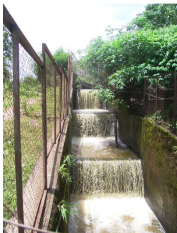
Figure 6.8 – Drop structure at Ban Nam Nyam
