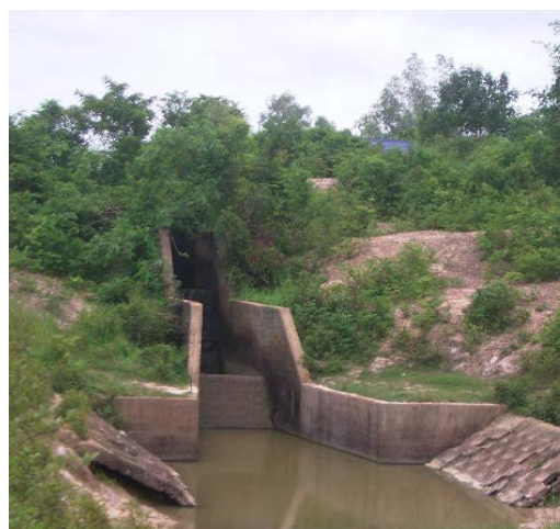
Figure 6.11 - Drop structure from downstream
