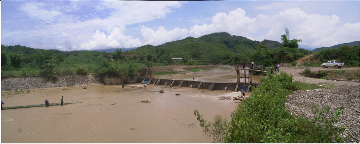
Figure 6.3. Nam Kay weir
