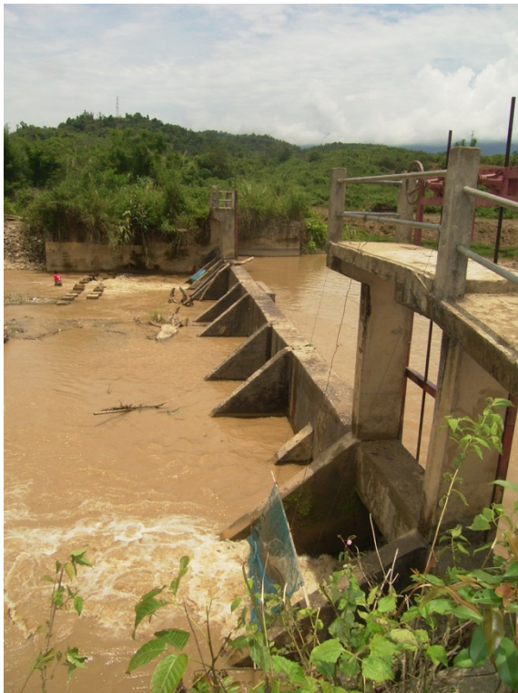
Figure 6.14. Nam Kay Weir and sluiceway
