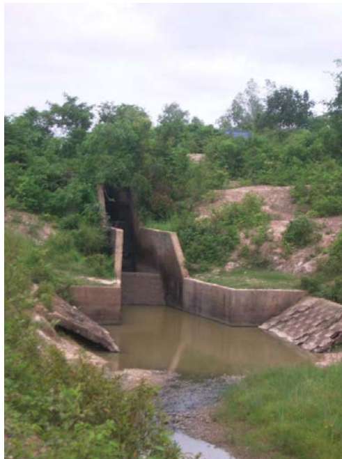
Figure 6.2. Drop structure on the Nam Houm irrigation channel
