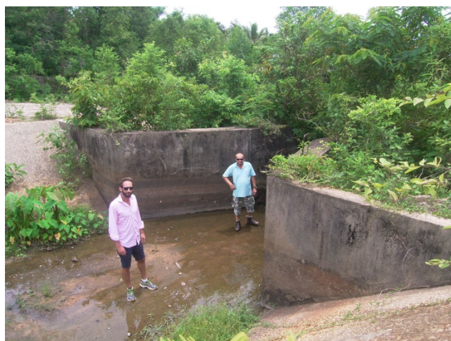
Figure 6.10. Entrance to drop structure
